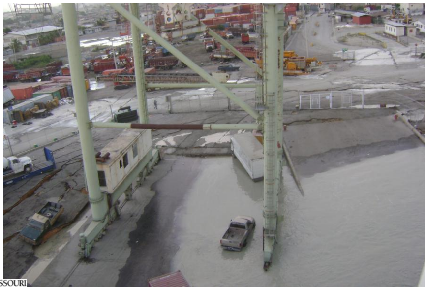
Liquefaction During 2010 Haiti Earthquake
