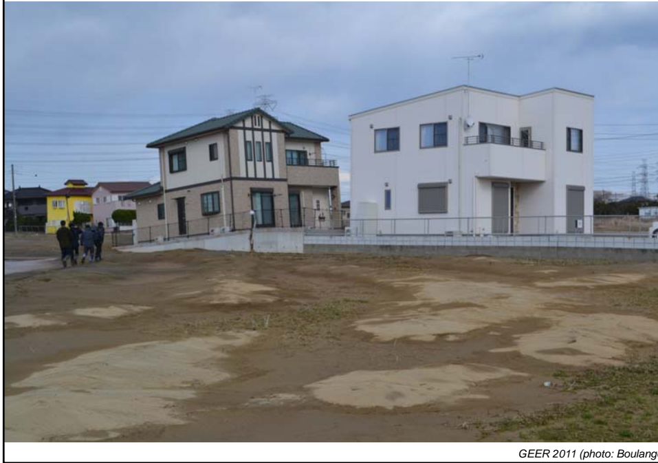
Effects on buildings (e.g., Kamisu City)
