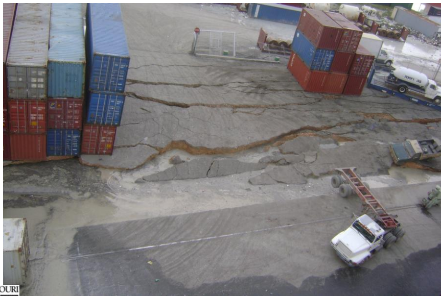
Liquefaction During 2010 Haiti Earthquake
